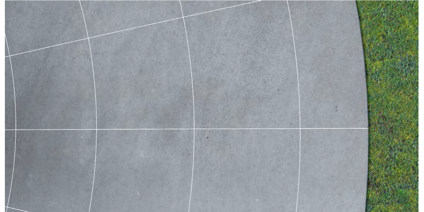
VERSION ( A ) Soft concrete surface with embedded aluminum profiles
